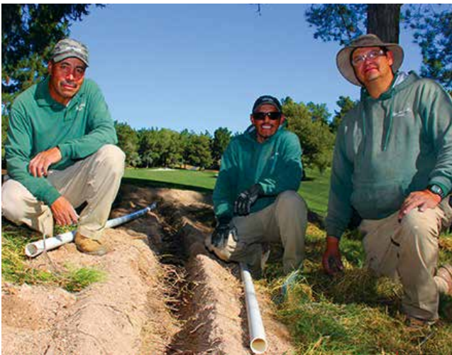
Shadow Creek irrigation manager Carlos Duran poses by a drip irrigation line recently installed around a tree. He and his team are surrounding nearly 7,000 trees throughout the golf course with similar drip line.
